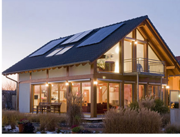
Home photovoltaic system
